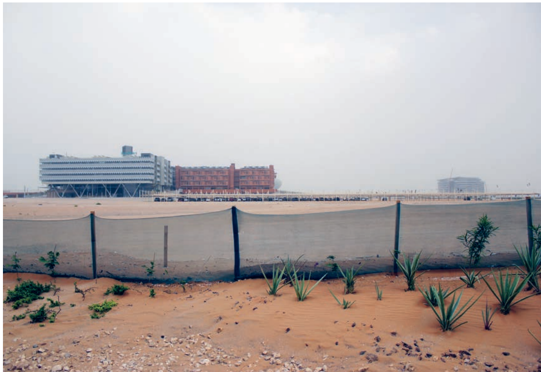
Masdar Institute, a graduate-level research center that focuses on renewable energy and clean technology, was designed by Foster + Partners. Photograph by Gökçe Günel, 2014.
