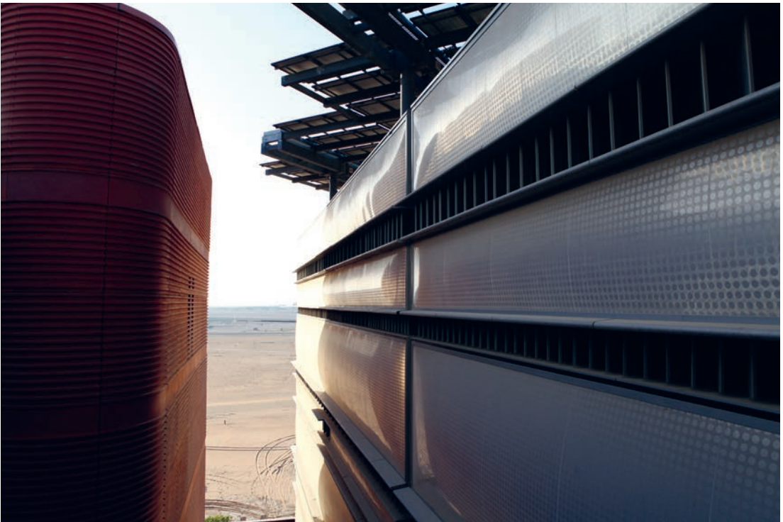
The laboratory façades at Masdar Institute are composed of insulating cushions that shade the interiors of the building and remain cool to the touch under the desert sun. Photograph by Gökçe Günel, April 2011.
