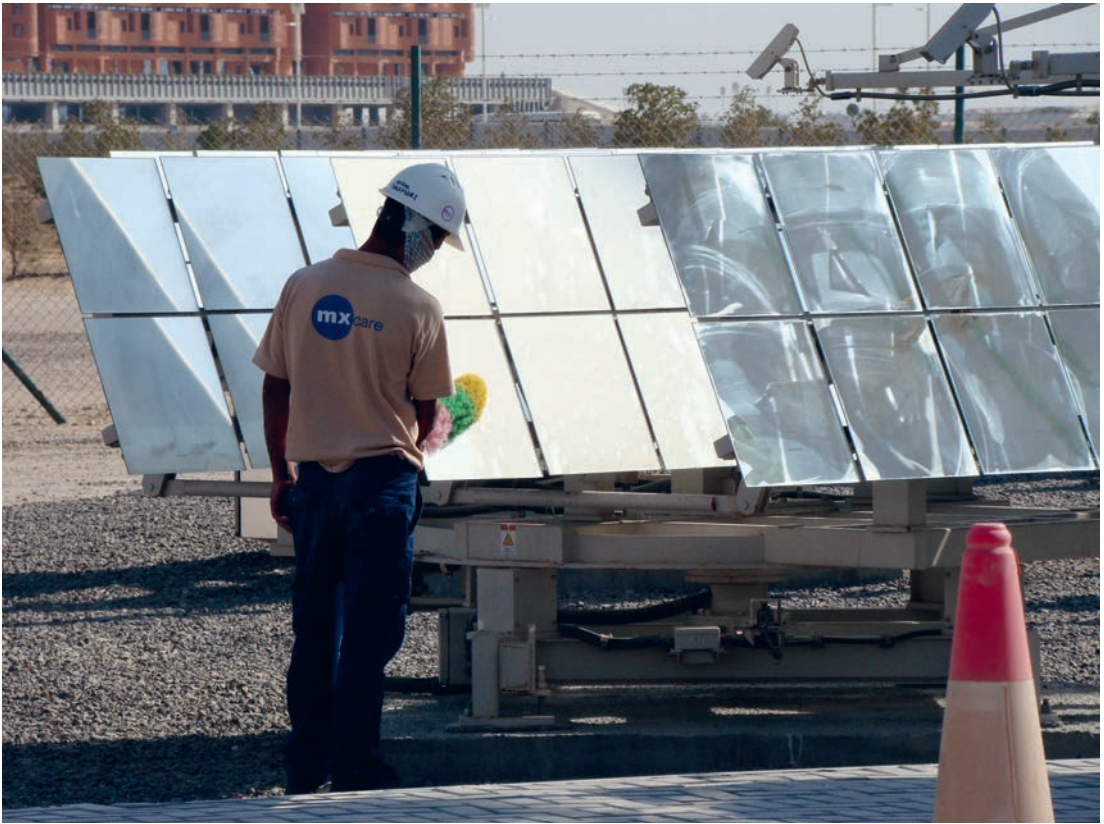
“Man with a brush” clears the thick coatings on solar panels, which result from a mixture of dust and humidity, and ensures their efficacy. Photograph by Gökçe Günel, April 2011.
