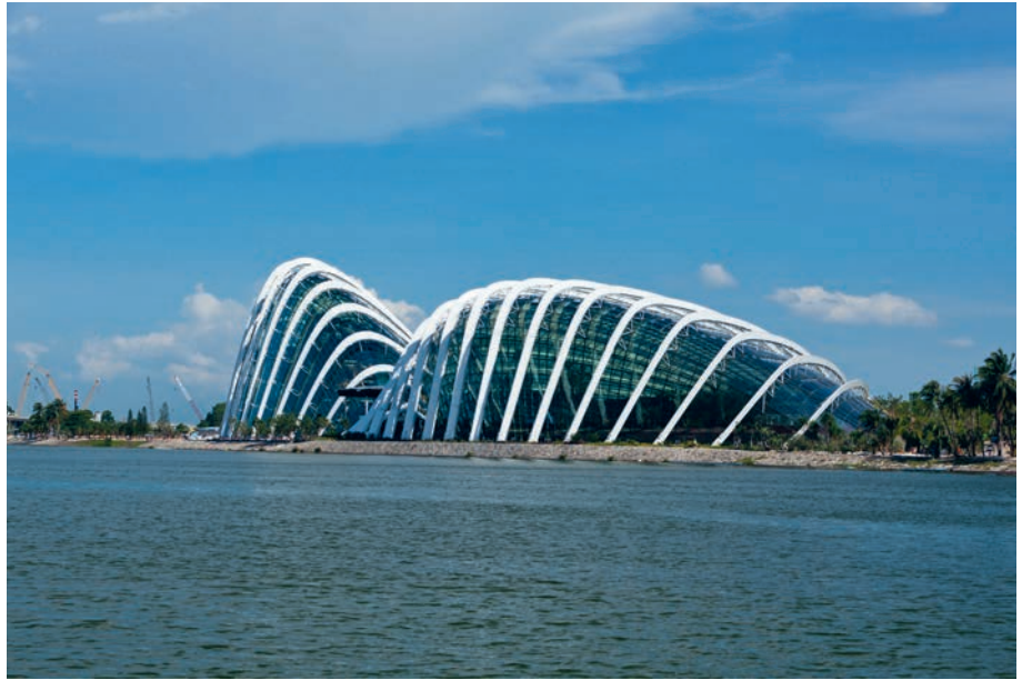
"Cooled Conservatories," Gardens by the Bay, WilkinsonEyre Architects, Singapore, 2006–2012. Courtesy of WilkinsonEyre.
