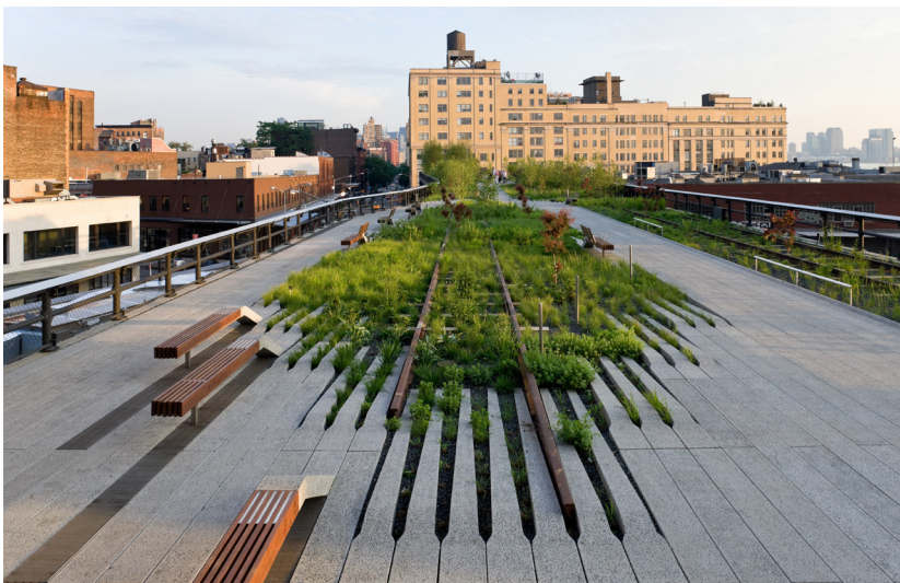
Field Operations and Diller Scofidio + Renfro, The High Line Park, 2006–2014. Photograph by Iwan Baan.
