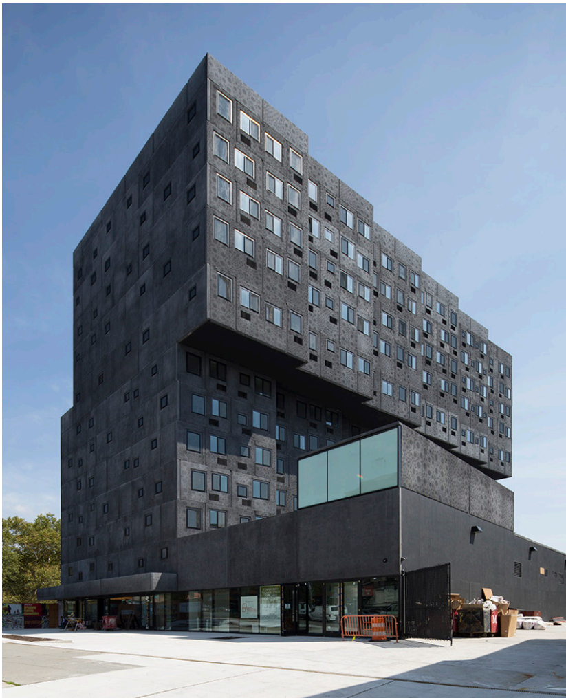
Exterior of the Sugar Hill Project, in which the building’s three separate entrances are located on Saint Nicholas Avenue. Photograph by Ed Reeve. Courtesy of Adjaye Associates.
