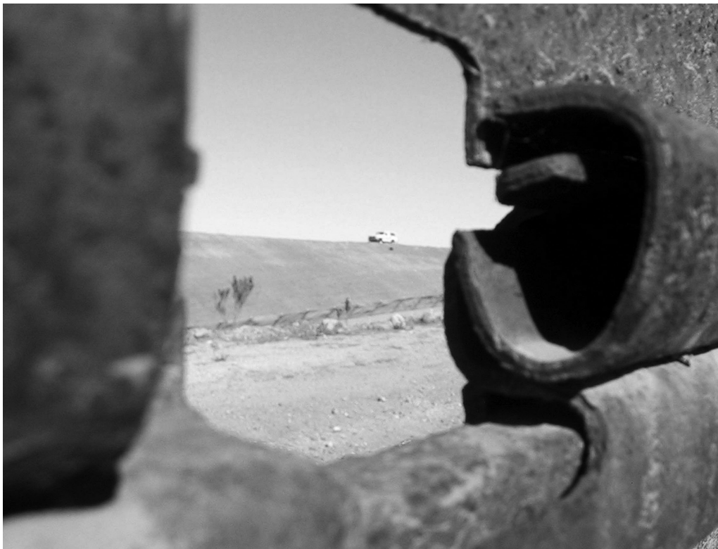
A current section of the US–Mexico border wall built in the 1990's with recycled temporary air-landing mats used in the desert storm war in the Middle East. Courtesy of Estudio Teddy Cruz + Forman.
