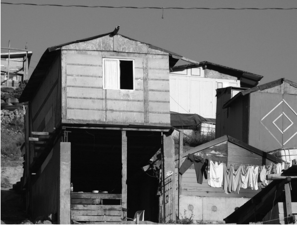
Informal settlements in Tijuana build themselves temporally with discarded houses, garage doors, and other debris from San Diego. Courtesy of Estudio Teddy Cruz + Forman.
