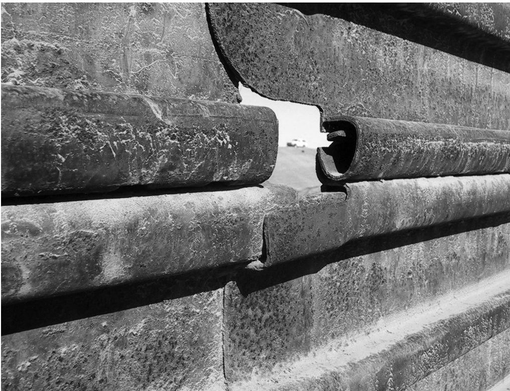
A current section of the US–Mexico border wall built in the 1990's with recycled temporary air-landing mats used in the desert storm war in the Middle East. Courtesy of Estudio Teddy Cruz + Forman.
