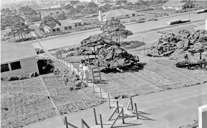
Two women walk along one of the many painted sidewalks next to a street sign that reads "Synthetic St." in the fake-townscape camouflage at Boeing Plant 2, 1941-1945. © Tom Philo.
