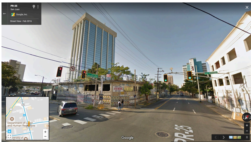
Department of Labor and Human Resources at the Prudencio Rivera Martínez Building. Courtesy of Google Street View.
