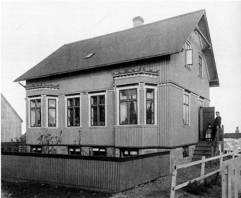
Vesturgata 18, Reykjavík, since moved to Bóklöðustígur 10. This is a very early version of a Corrugated Iron Sweiser, an Icelandic adaptation of the Norwegian Sweiser. Originally published in Hörður Ágústsson, Íslensk Byggingarfléið I: Ágrip Af Húsagerðarsögu 1750–1940 [Reykjavík: Húsafríðunarnefnd ríkisins, 1998], 112.
