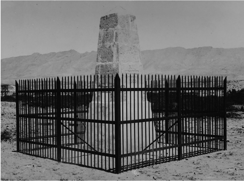
Monument No. 1 fortified with an iron fence. From the International Boundary Commission survey of 1891–1896. Photograph by J. H. Wright, US National Archives [77-MB-1-1].
