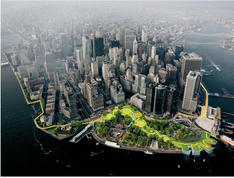
“The Big U,” proposed by BIG [Bjarke Ingels Group] with One Architecture, Starr Whitehouse, James Lima Planning + Development, Green Shield Ecology, AEA Consulting, Level Agency for Infrastructure, ARCADIS, and Buro Happold. Courtesy of BIG.
