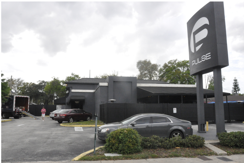
When this photo was taken, the nightclub had recently been painted a dark charcoal color and the unpermitted fence was painted black. Photo of Pulse taken by the City of Orlando as part of a fire inspection and occupancy load evaluation conducted on March 11, 2015. Courtesy of City of Orlando.
