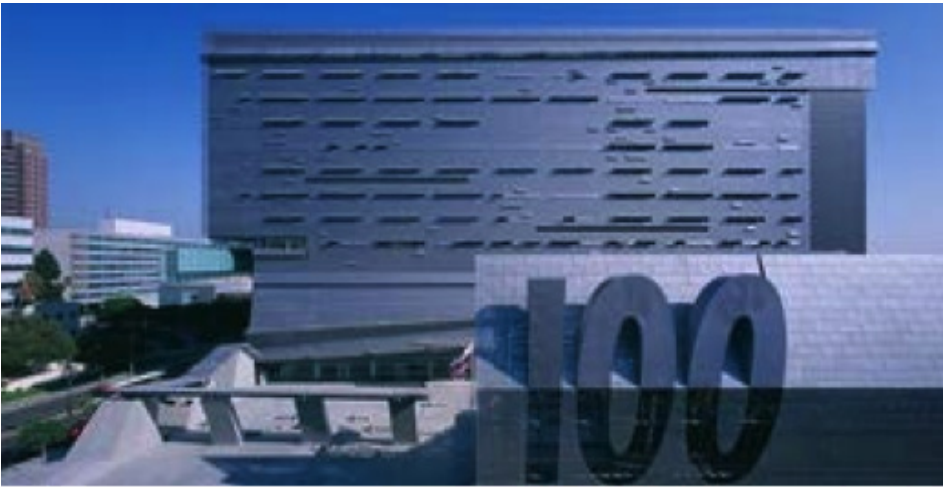
Morphosis Architects, Caltrans District 7 Headquarters, 2004. Image from: Clark Construction, http://www.clarkconstruction.com/our-work/projects/caltrans-district-7-headquarters .
